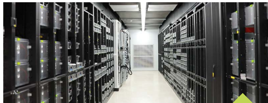
Hot aisle: Hot air evacuation and air pressure, temperature, and humidity monitoring
